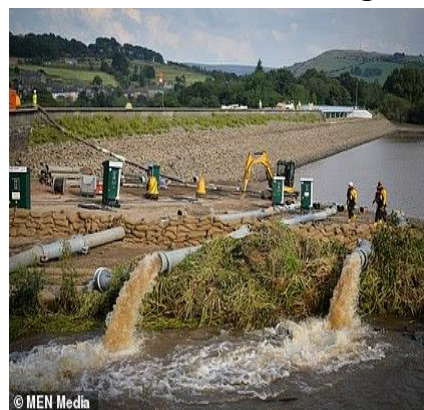
Pumping water from the reservoir
